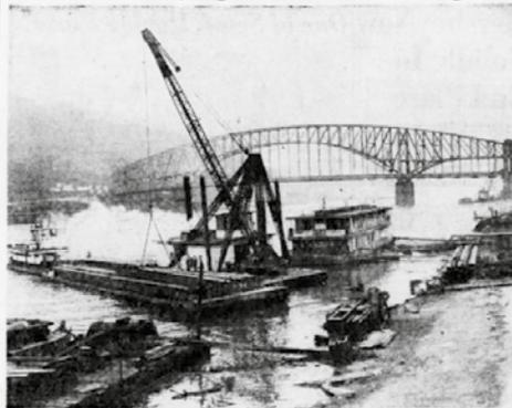
PILE DRIVING — Activity at Pittsburgh's changing Point increased yesterday when more barges and derricks moved in to begin driving piles for the sub-structure of the new Fort Pitt Bridge across the Monongahela River. The bridge, another link in the Penn-Lincoln Parkway, is to be located about 200 feet east of the Point Bridge. Construction of trestle piers on the Monongahela and Allegheny River banks, by the Dravo Corporation, is advancing rapidly.
