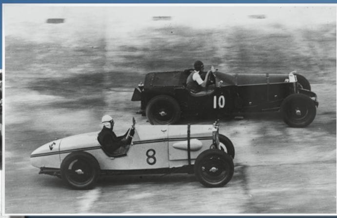
Post-Vintage spirit - pounding round the uneven Brooklands Outer Circuit banking, MG NE versus Invicta. The NE used an overhead camshaft 1271 cc 6-cylinder engine
